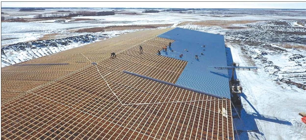
Work on the roof of the massive new hog finishing barn at the Plainview Colony. The massive building measures 172 feet by 710 feet. It will ship out 700 hogs a week to the Maple Leaf plant at Brandon. See inside for more photos.
