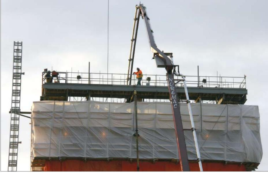
Workers on the top deck above the slipform as concrete is pumped into the form. Workers up top place rebar and finish the concrete as the slipform rises.
