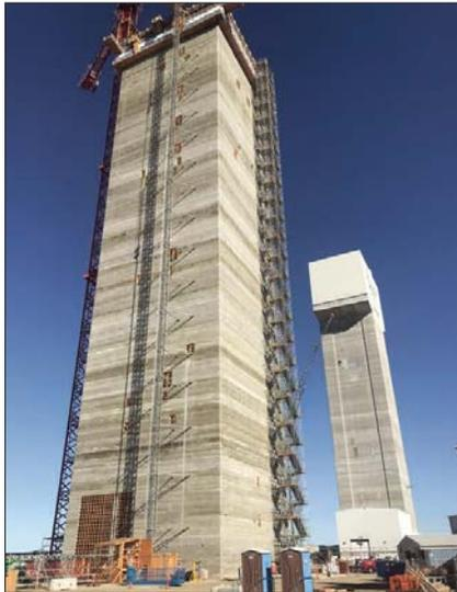
The continuous pour on the south headframe at K3, part of the \$3 billion expansion of Mosaic Esterhazy's K3, was completed on September 4—three days ahead of schedule. At 380 feet, the north headframe at right in the photo is the tallest structure in Saskatchewan. Crushrite Concrete provided the concrete for the pour.
