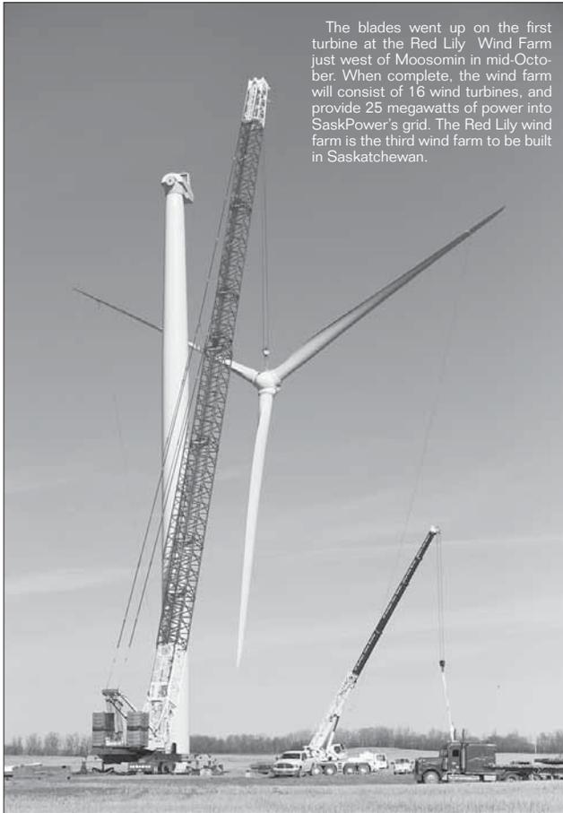
The blades went up on the first turbine at the Red Lily Wind Farm just west of Moosomin in mid-October. When complete, the wind farm will consist of 16 wind turbines, and provide 25 megawatts of power into SaskPower's grid. The Red Lily wind farm is the third wind farm to be built in Saskatchewan.
