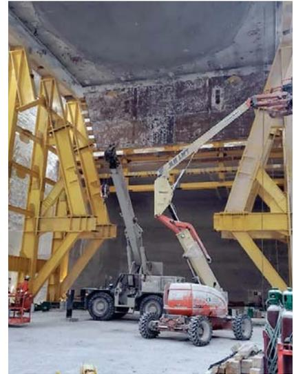
North coarse ore bin steel installation at K3.
