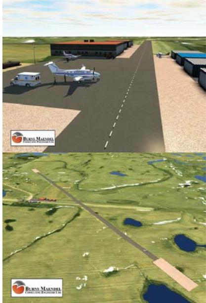
These renderings by Burns Maendel Consulting Engineers show the proposed expansion of Moosomin's airport. The new runway would run northwest-southeast in line with the prevailing winds. A new access road, taxiway, and apron would be built on the road allowance that the current runway is built on.
