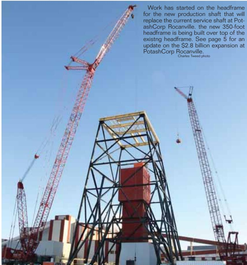
Work has started on the headframe for the new production shaft that will replace the current service shaft at PotashCorp Rocanville. The new 350-foot headframe is being built over top of the existing headframe. See page 5 for an update on the \$2.8 billion expansion at PotashCorp Rocanville.
